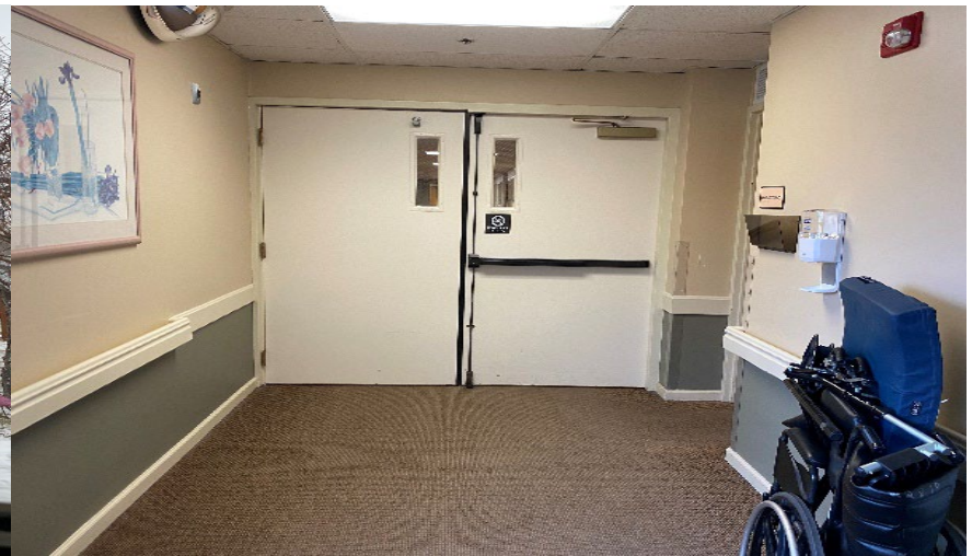
Fire Door Separating the Assisted Living from the SNF
